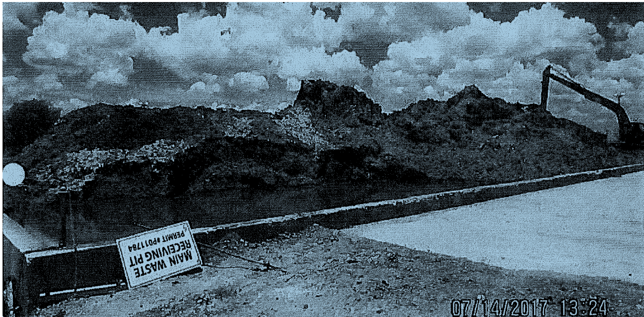
A 2017 Railroad Commission inspection photo of DeWitt's overloaded main waste pit in Cuero.
